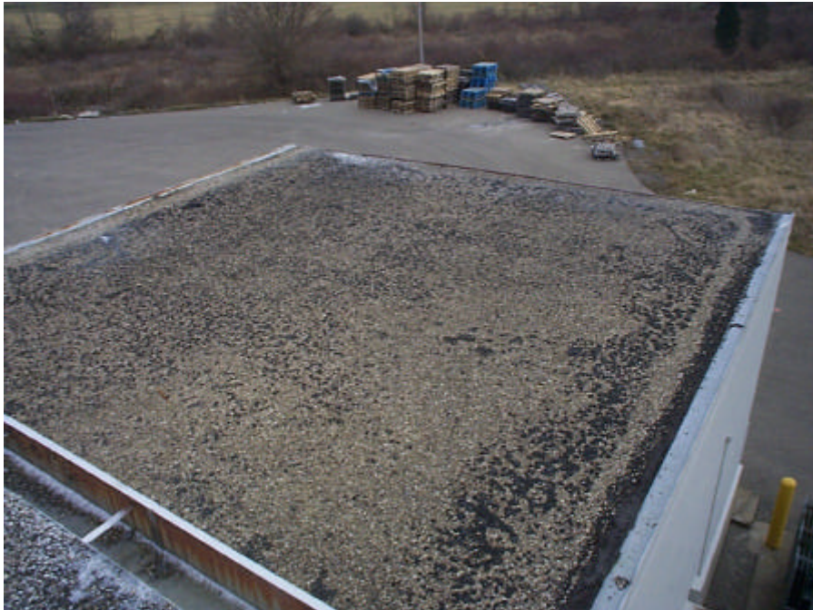
PHOTOGRAPH 4 View of east roof over loading dock area.
