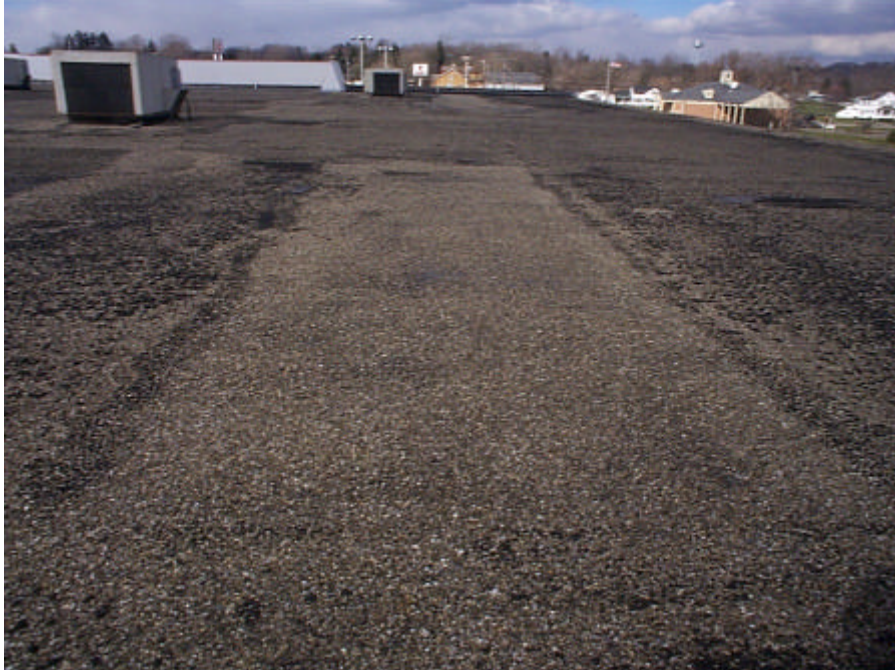
PHOTOGRAPH 3 Main roof overview looking northeast.
