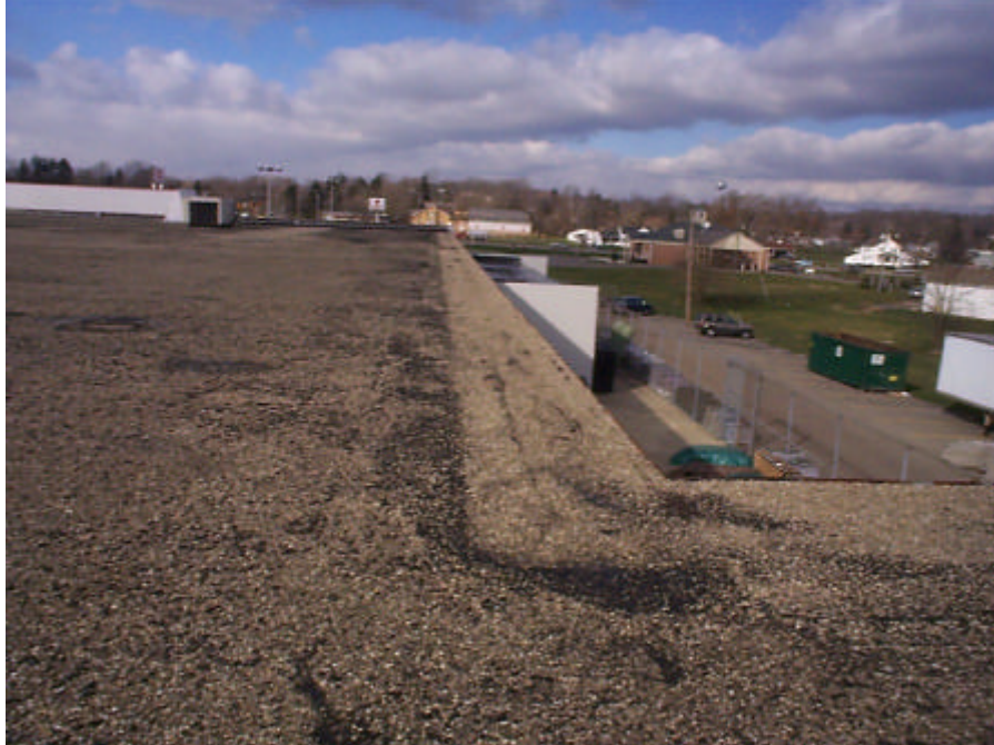
PHOTOGRAPH 13 Edge repairs along north side of main roof.
