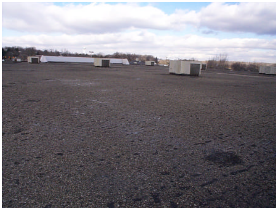
PHOTOGRAPH 2 Overview of main roof area looking northwest from southeast corner.
